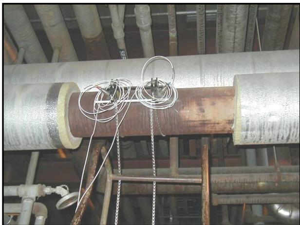
**Figure 4 - Ultrasonic Flow Cells on the Discharge Piping**
