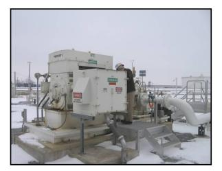
Figure 5 – Main Line Pumping Unit (MLPU) 8X10X13-3 Stage Pump
