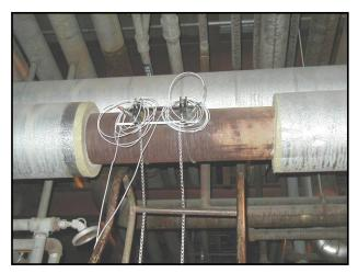
Figure 4 - Ultrasonic Flow Cells on the Discharge Piping
